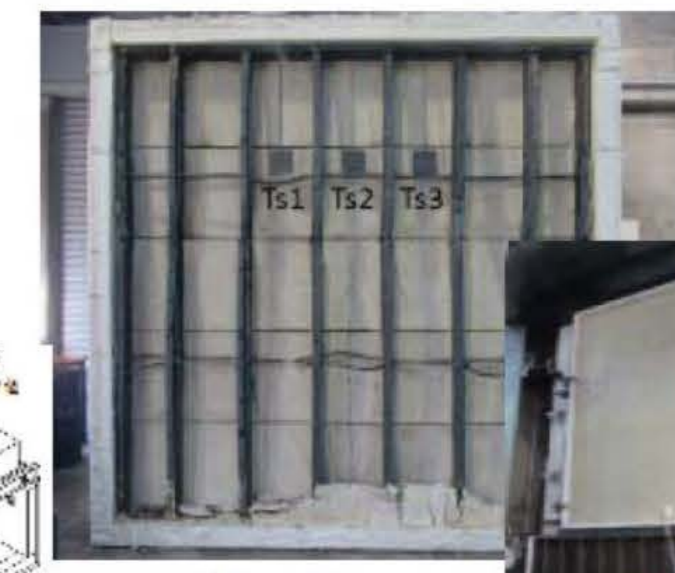
Fire Compartment Wall
