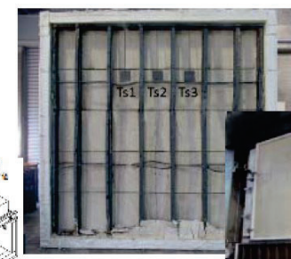
Fire Compartment Wall
